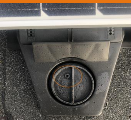
Bayonet safety pin location
