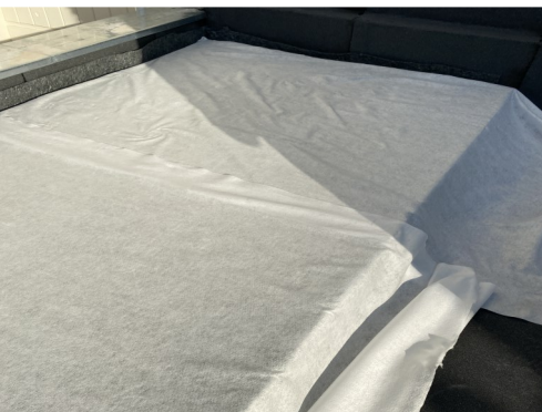
Encapsulate the cells with FV 125 fleece
