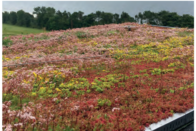
Sedum roof (BauderEXTENSIVE LIGHTWEIGHTsedum)
