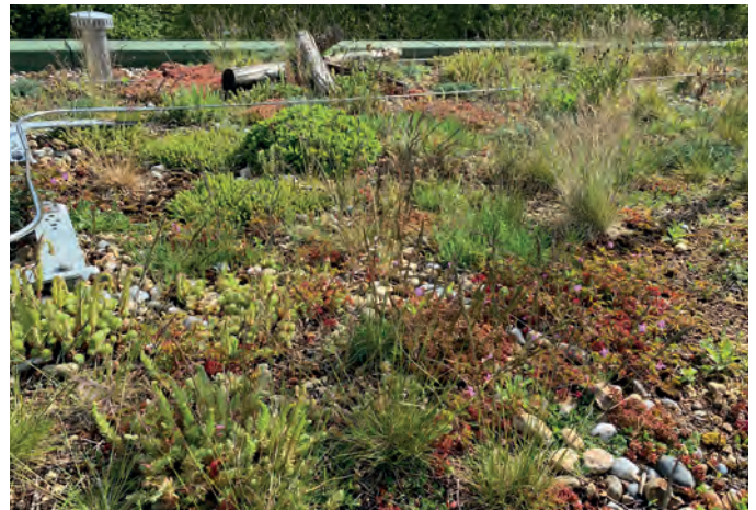
Biodiverse roof (BauderGREEN Plugs and BauderGREEN Flora 5 Seed Mix)
